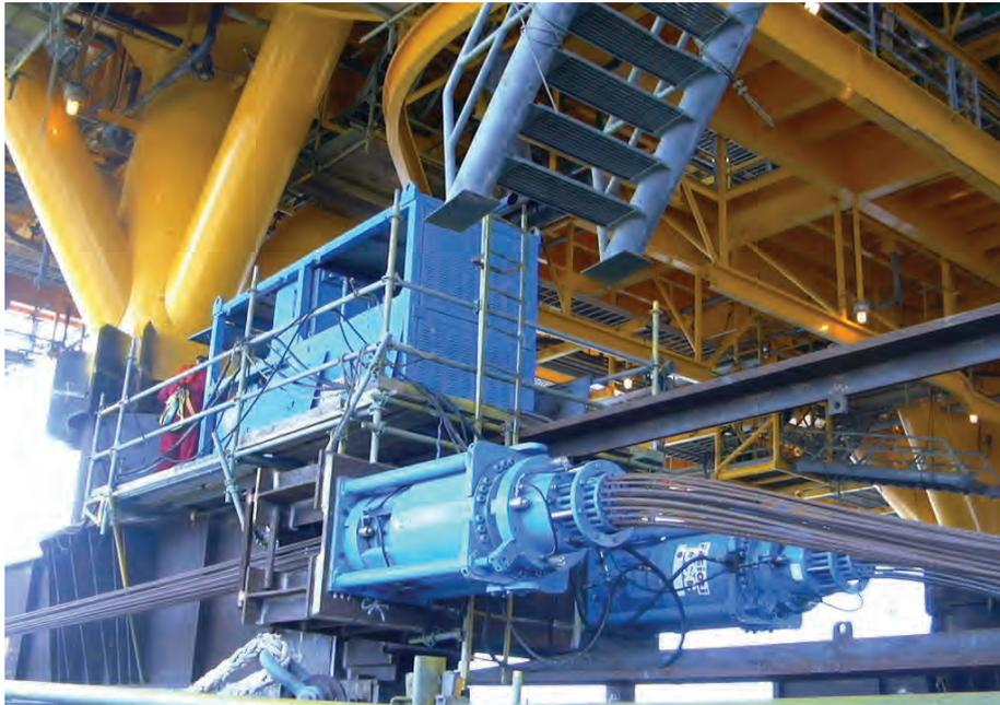
uncommon) on a small footprint. The small footprint causes less site disturbance than a crane of equal capacity. The cost of shipping strand jacks around the world is small compared to a crane.
