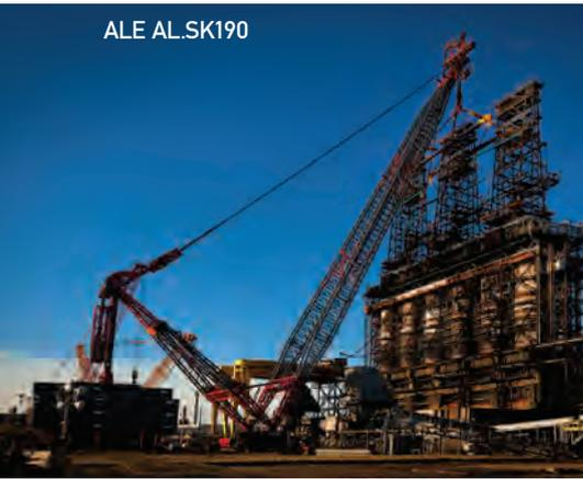
the radius would be increased by 5 m as the boom from where the lift takes place sits on the ring. This creates the illusion that the crane is stronger than it is. In addition, a larger ring diameter (with the rest of the crane components remaining equal) would result in a larger radius and could wrongly lead someone to believe that the crane has increased in capacity.
