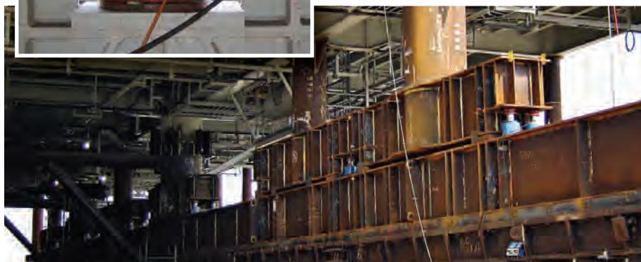
FIGURE 5 Multiple Versabar load cells and jacks per strong point
