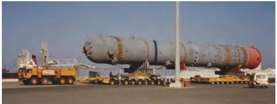
This article assumes that the decision to use turntables has already been made and that the transport has already taken place to the final destination. The transporters are in their offload locations and the cranes, a main crane and a tailing crane, are in position and hooked up to the vessel. The lift is about to commence.
